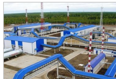
Oil Pump Station "Tayezhnaya", Transneft
